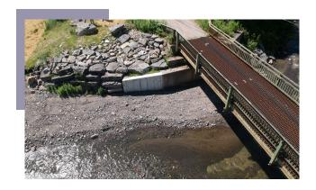
In July 2024, the Town of Newport completed the restoration of the Woodchuck Hill Road Bridge in partnership with Slate Hill Constructors, Inc. and Plumley Engineering, P.C. Woodchuck Hill Road Bridge had damaged abutments and wing walls, which were removed and replaced with new retaining walls and riprap embankment erosion details.
